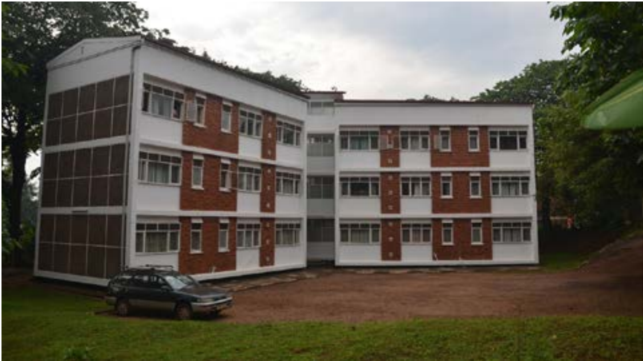
An exterior view of Mugenyi Flats.
